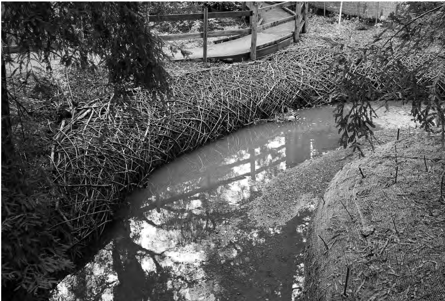
As part of the “Shaped by Water” exhibition, community volunteers built this willow sculpture at Adobe Creek in Los Altos in January. Designed by Daniel McCormick and Mary O’Brien, the sculpture is designed to help nature rebuild the eroded bank over time.
